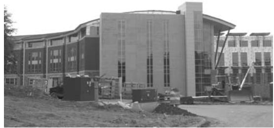
Figure 9.3 The new Lowes Corporate Headquarters under construction, 2003, Calloway Johnson Moore and West, architects. This refreshingly contemporary design is free from the needless neoclassical ornamentation so beloved by other North Carolina architects.
